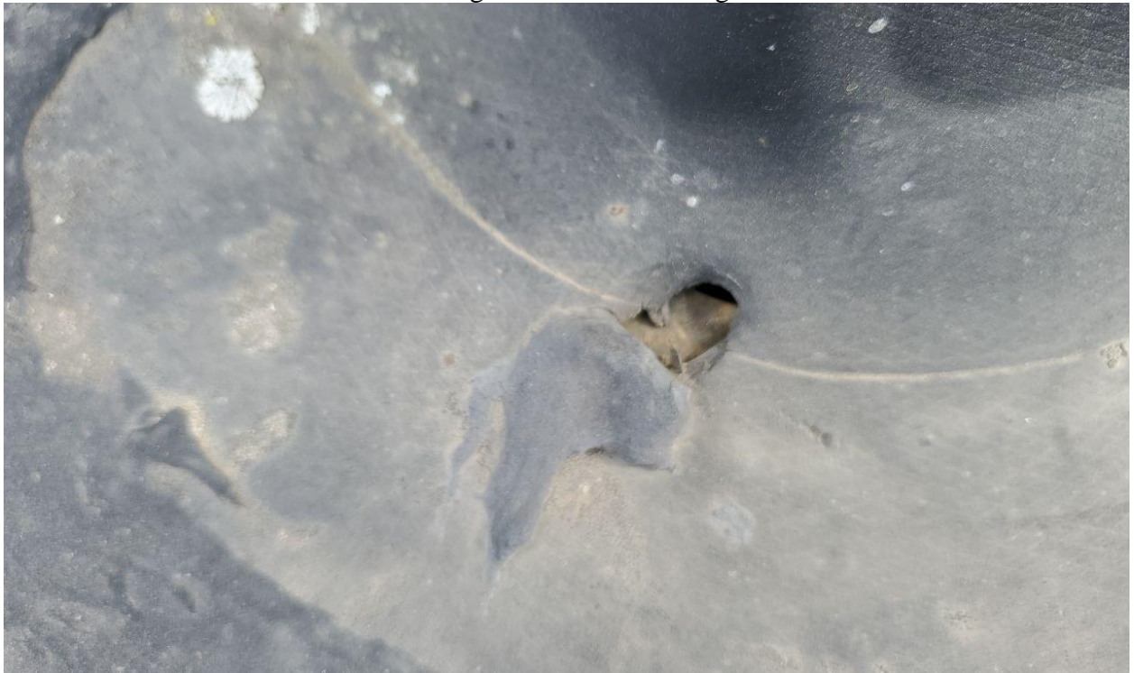
Failing Penetration Flashing
