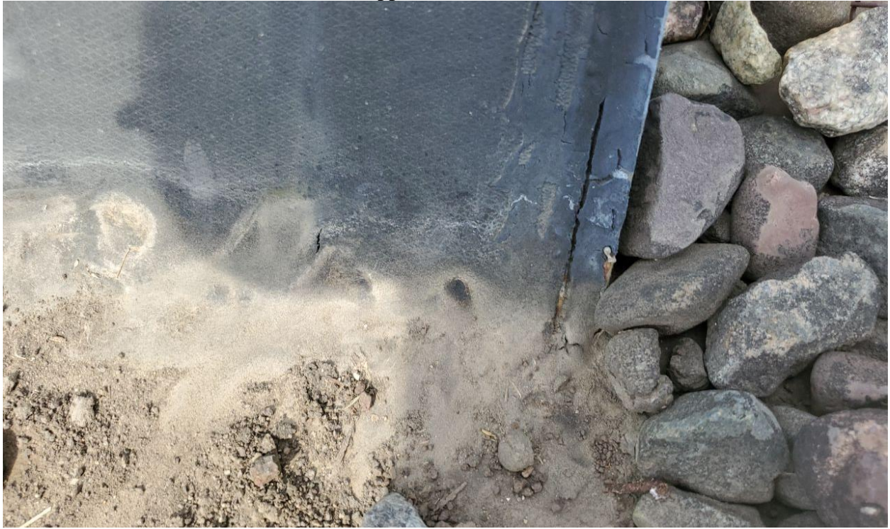
Scupper-Drain Failure
