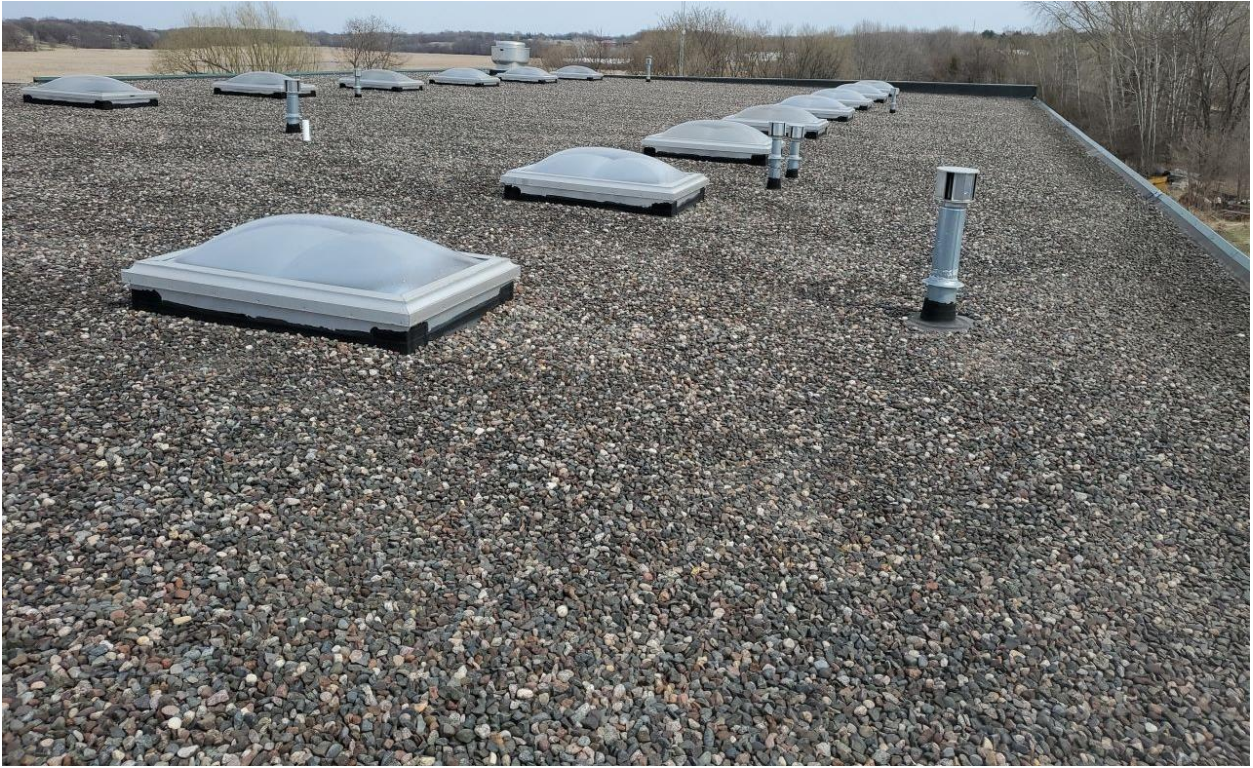
Overview of Roof
