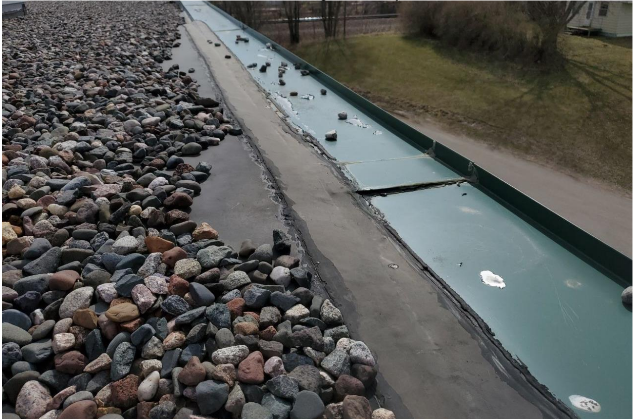
Metal Flashing Deficiency
