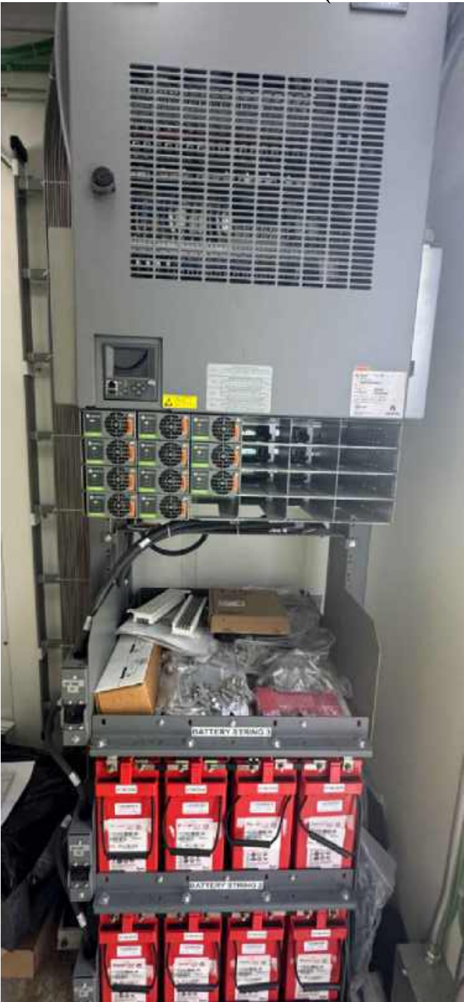
(E) AT&T NETSURE 7100 POWER PLANT W/(11) -48V RECTIFIERS & (8) 190AH BATTERIES
