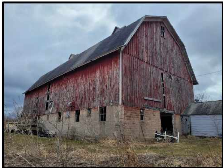
Figure 9: Barn on Southern Edge of the Property Facing Southeast.
